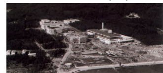
Scene during construction of Komagane Plant
